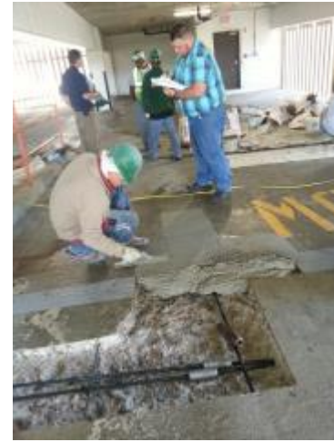
Post tension cable (PT cable) that had to be repaired on the surface in the East garage
