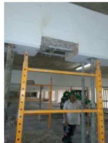
Overhead beam under repair in the garage
