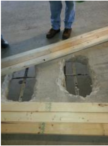
Post tension cable (PT cable) that had to be stretched and repaired in the East garage
